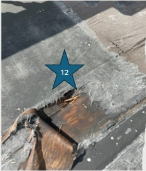
2 nd Level Deck Deterioration
